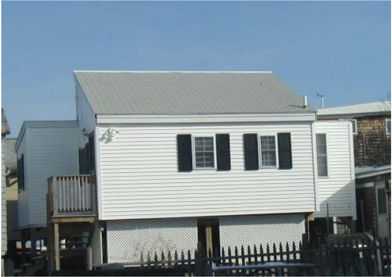
OUTSIDE, VIEW 1 from Eastern Ave.
